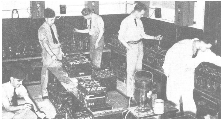
Just playing around in the Battery Room.
