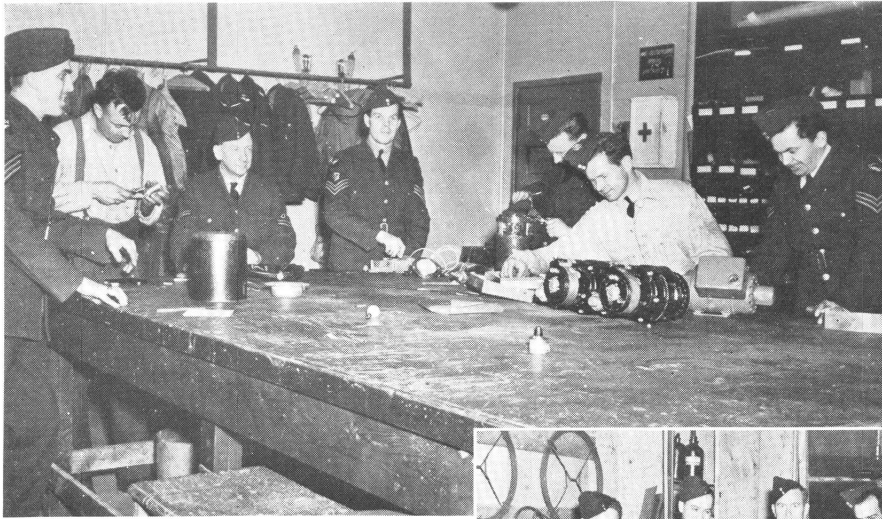
This group of electricians keep the electrical installations humming with life.
