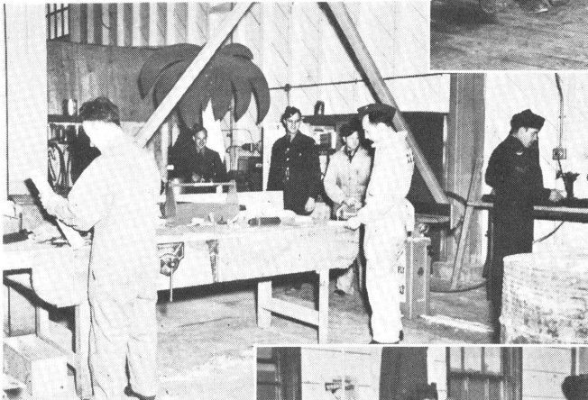
This happy gang are the plumbers. They are kept active repairing and servicing the huge sewerage system on this station.
