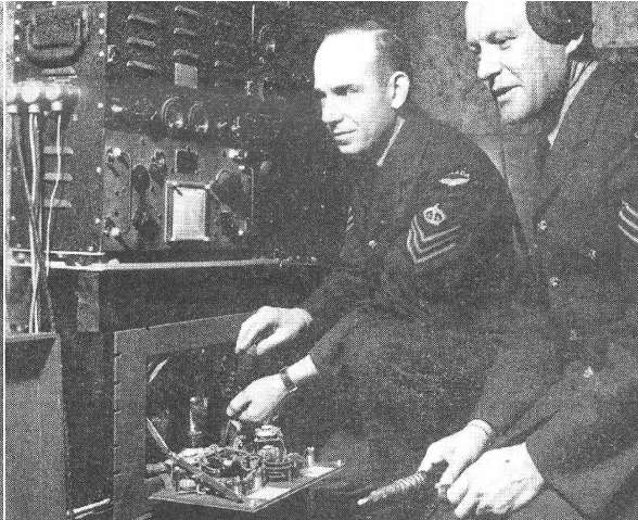
F/S. F. E. Anderson, chief engineer of G.B.S., is shown at the transmitter perfecting some flaw as Sergeant H. J. Christensen checks to see that the tone is improved.
